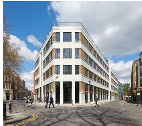
The Buckley Building 85,000 sq ft
