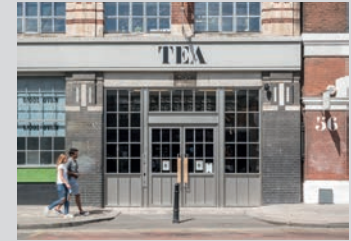
Tea Building E1
