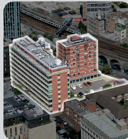
230 Blackfriars Road SE1 Redevelopment Start date: 2030+
